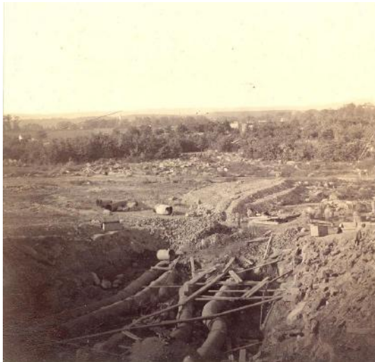
Figure 6. Buried Pipes in Connection with the New Reservoir, c.1862. vi
